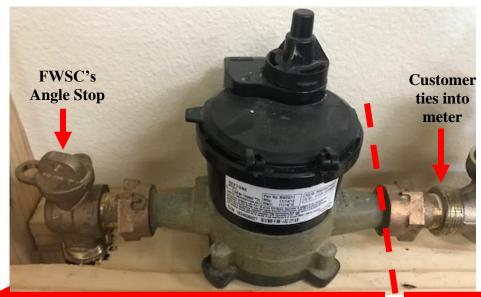
**Customer** is required to install a personal cut off valve about two feet after the meter.
